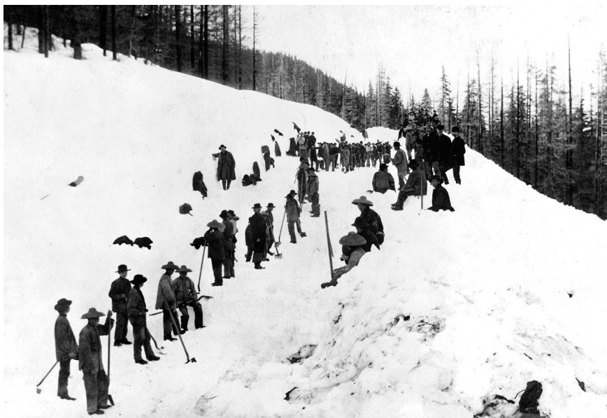
Chinese workers clearing snow from railroad tracks near the summit of the Cascades, 1886. Courtesy of the University of Washington Libraries, Special Collections, SOC0049.
